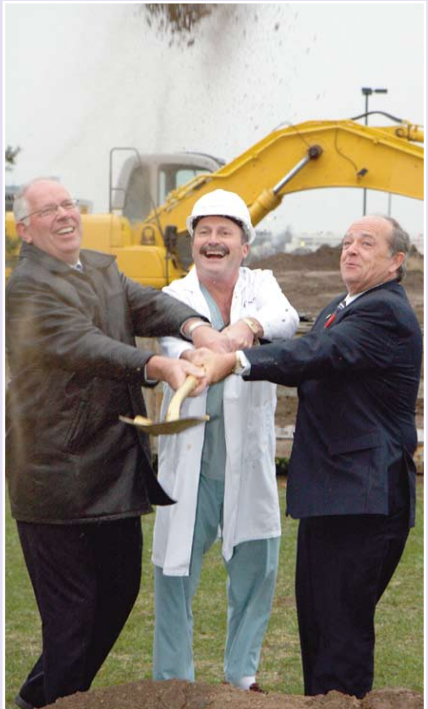
John Wiersma, Chair of the Foundation's Board of Directors, left, tosses a ceremonial shovel of dirt with Dr. Tom Stavro Sholdoff, Program Chief of Emergency, and Durham Regional Chair Roger Anderson at the November 2007 groundbreaking of the Rouge Valley Ajax and Pickering redevelopment project.
